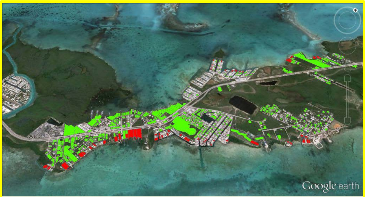
Figures 9a and 9b. Action 1 Scenario: Images of two (2) locations in Key Largo area. Parcels in red indicate those that are located in a FEMA V-Zone and had their buildings elevated (189 total) as a result of the candidate action. Parcels in green indicate those that are located in a FEMA A-Zone and had their buildings floodproofed (2283 parcels total) as a result of the candidate action.
