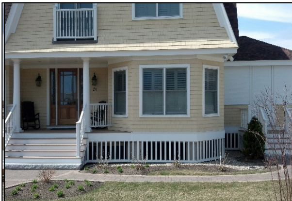
Figures 8a and 8b. Elevated house (left) and floodproofed house (right). Source: http://www.theepochtimes.com/n3/4747-hurricane-sandy-katrina-offer-similar-lessons-for-builders/
