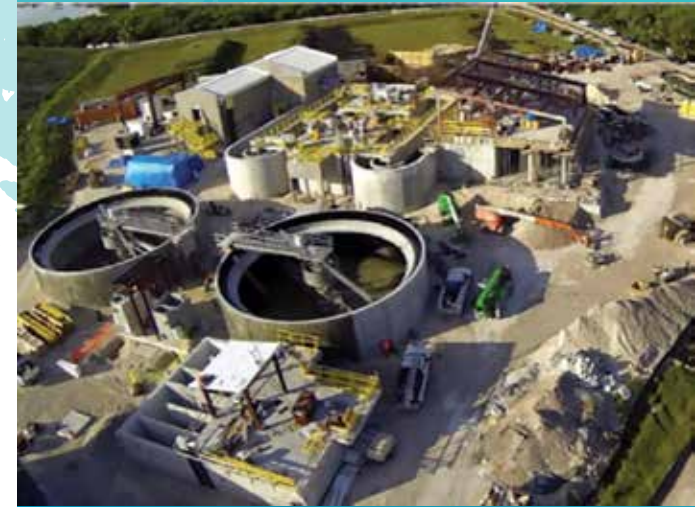
Construction of Cudjoe Advanced Water Reclamation Facility
