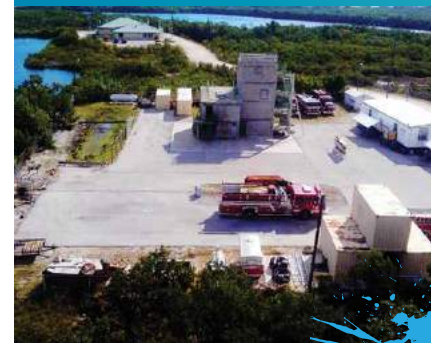
Crawl Key Training Academy Capital Project PHOTO SOURCE: Monroe County Emergency Management
