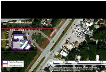
Building footprint digitization of the Murray E. Nelson Government Center PHOTO SOURCE: Monroe County, FL GIS Vulnerability Assessment for Sea Level Rise Planning
