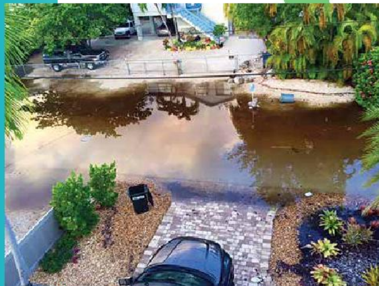
Nuisance Flooding, Key Largo, FL
