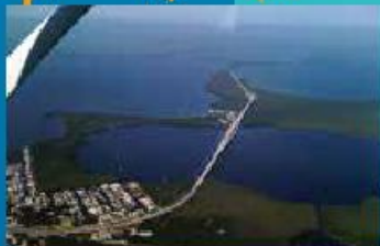
Aerial view of Jewfish Bridge with 18 mile stretch in the background and Key Largo in the foreground
